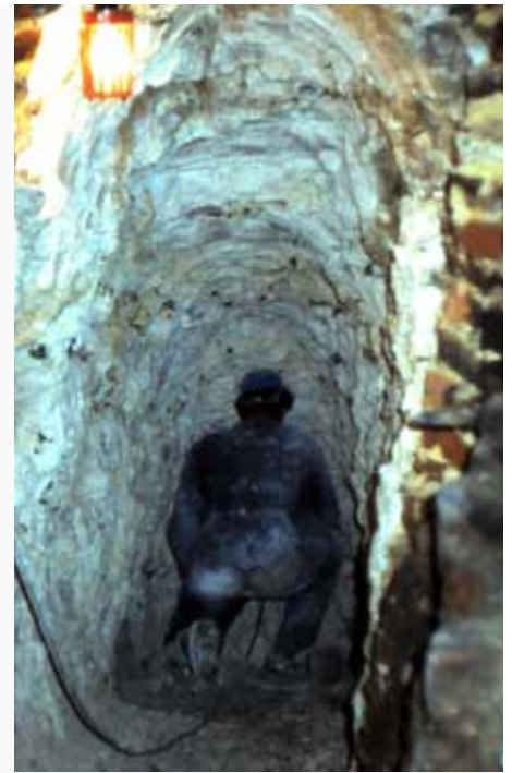
Fig.1 Construction of the world's first artificial cave in solid rock for hibernating bats
