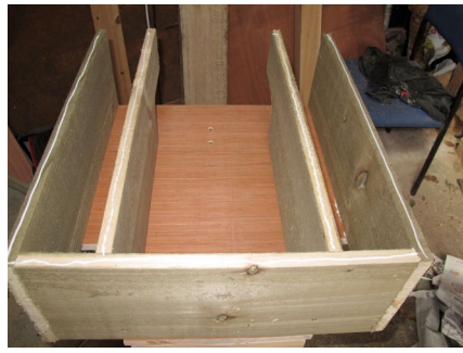
11. Run a line of wood glue along the edges of the walls and base.
